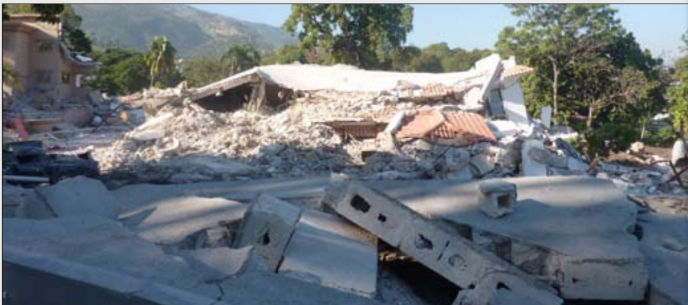
Buildings throughout Port-au-Prince and beyond lay flattened by the 7.0 earthquake.
