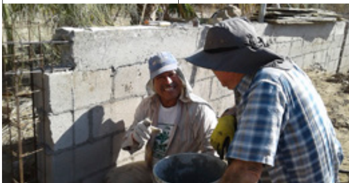
Darayl Larsen visits with the job supervisor.
