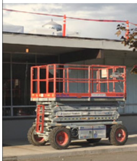
Roof work is under way on the building.
